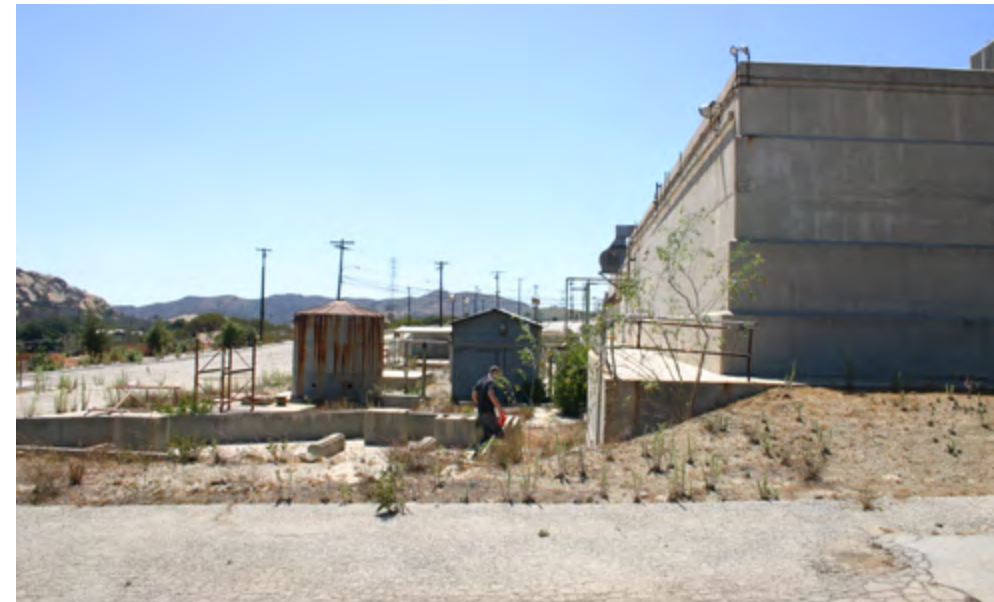
ELV STEPPED CONCRETE WALL SOUTHEAST EDGE
