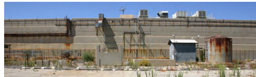
ELV WALL SOUTH FACE
