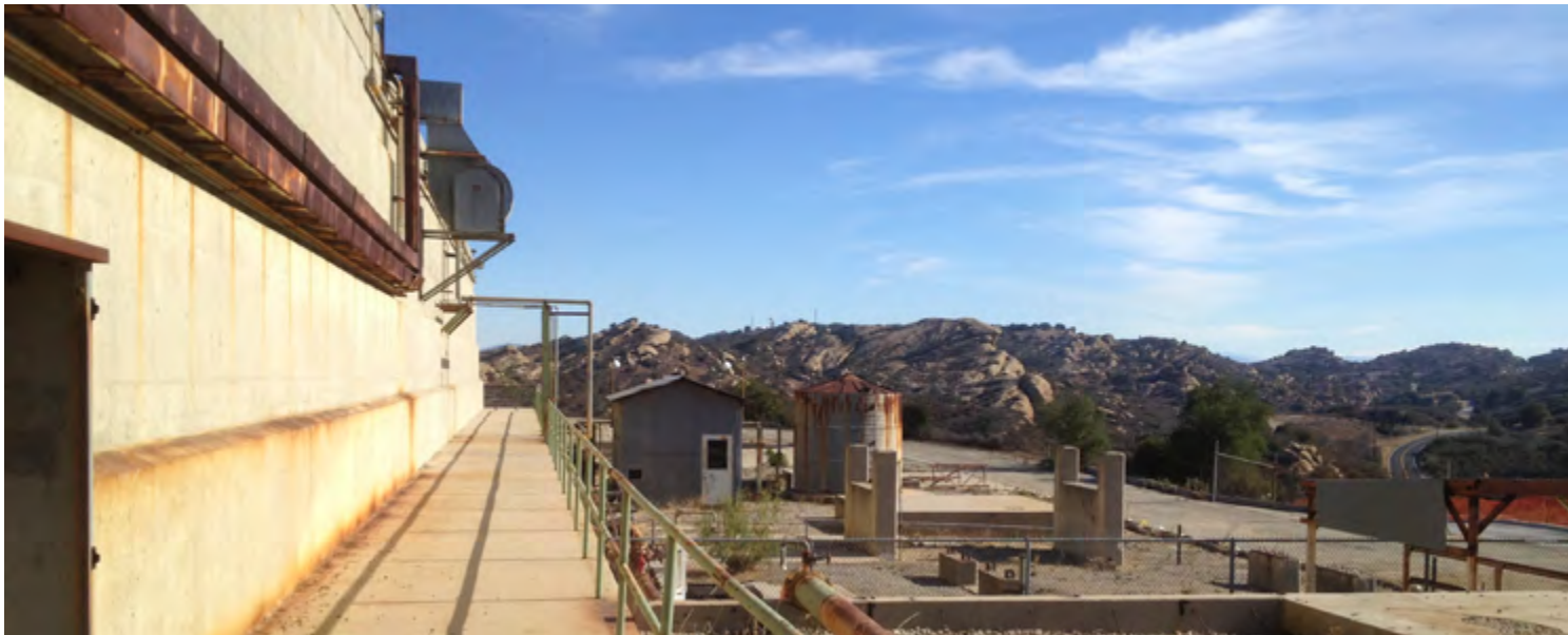
ELV WALL EXTERIOR WALKWAY
