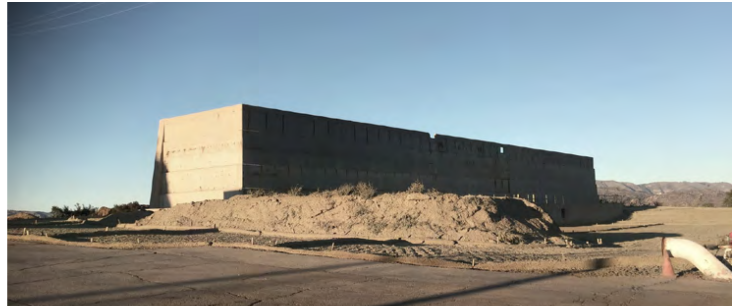
VIEW FROM SOUTHWEST OF ELV STRUCTURE WALL
