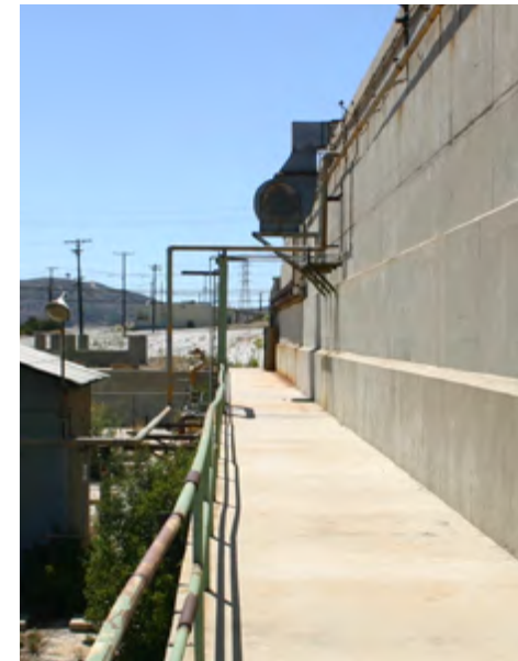
ELV WALL SOUTH FACE
