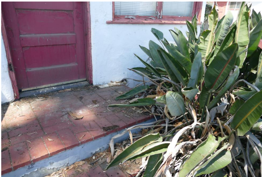
Figure 64. Tiled entry steps at Unit 7. Photo taken facing north.
