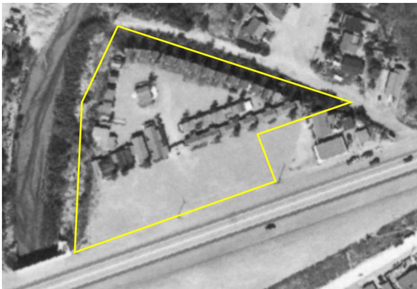
Figure 36. Aerial of the site from the 1940. (Source: Rosi Dagit, permission pending)
