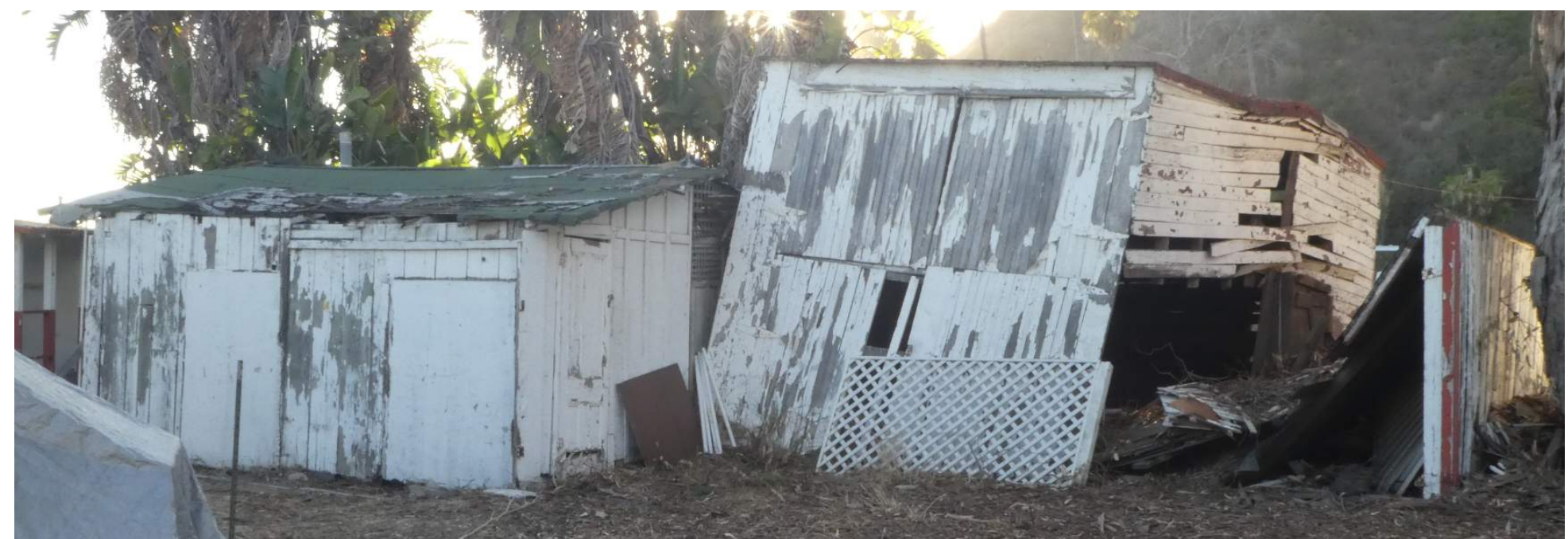
6 Barn & Shop East Elevation
