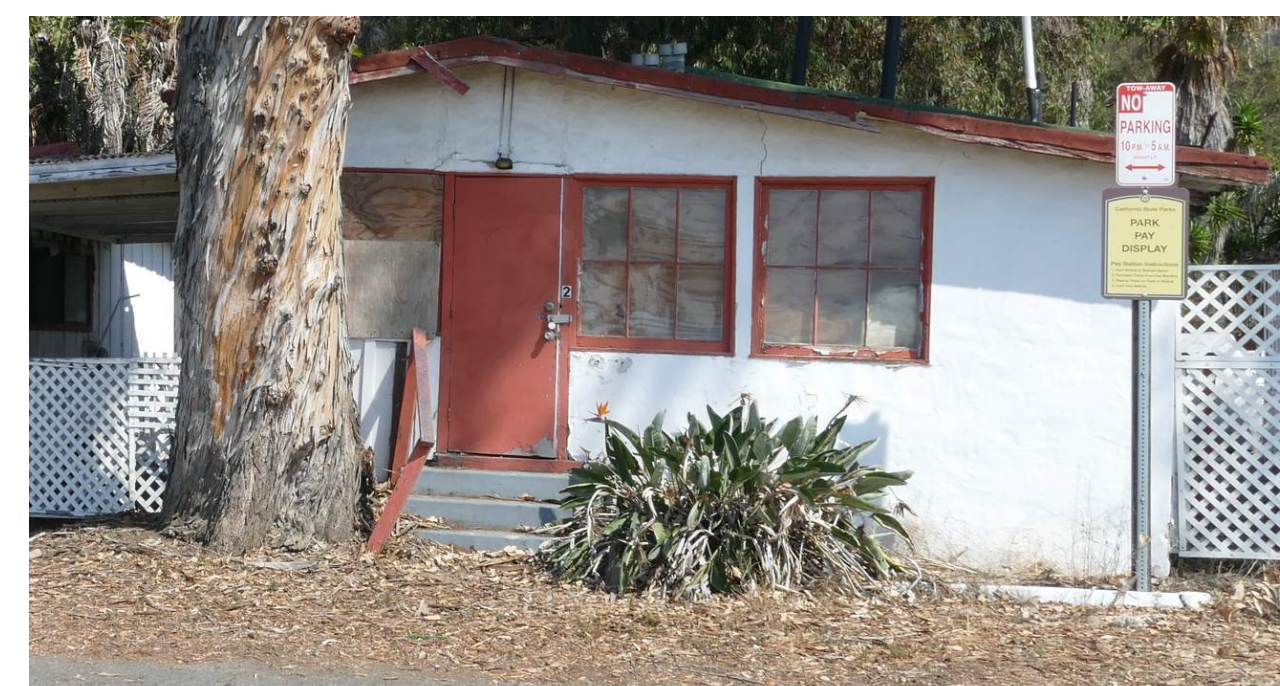
5 Unit 2 South Elevation
