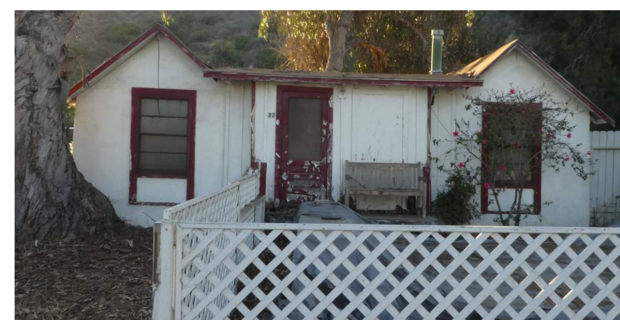
7 Unit 22 East Elevation
