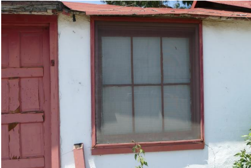
Figure 57. Typical multi-lite fixed wood window. Photo taken facing north at Office.
