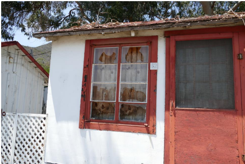
Figure 62. Typical casement steel window. Photo taken facing northwest at Unit 12.
