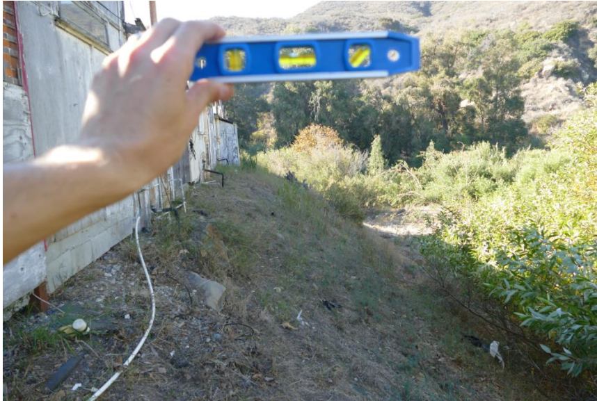
Figure 15. Northeastern embankment with an approximate slope of 30°. Photo taken facing northwest.
