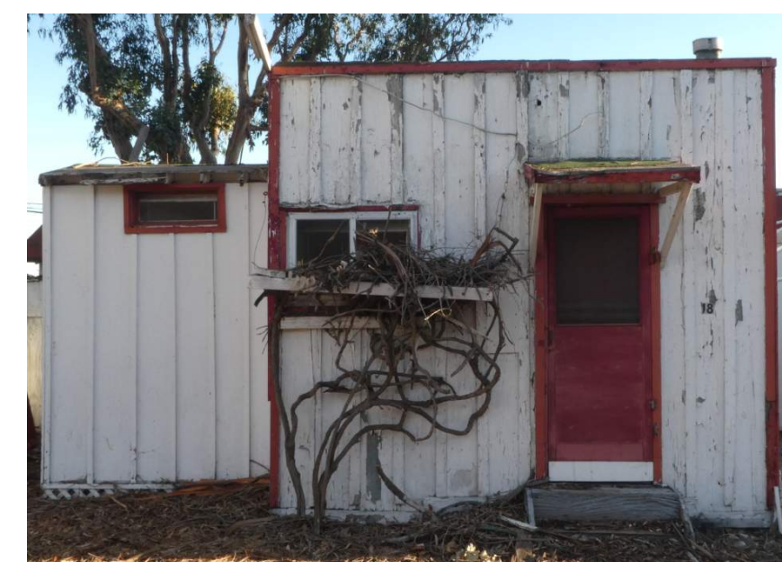
8 Unit 18 North Elevation
