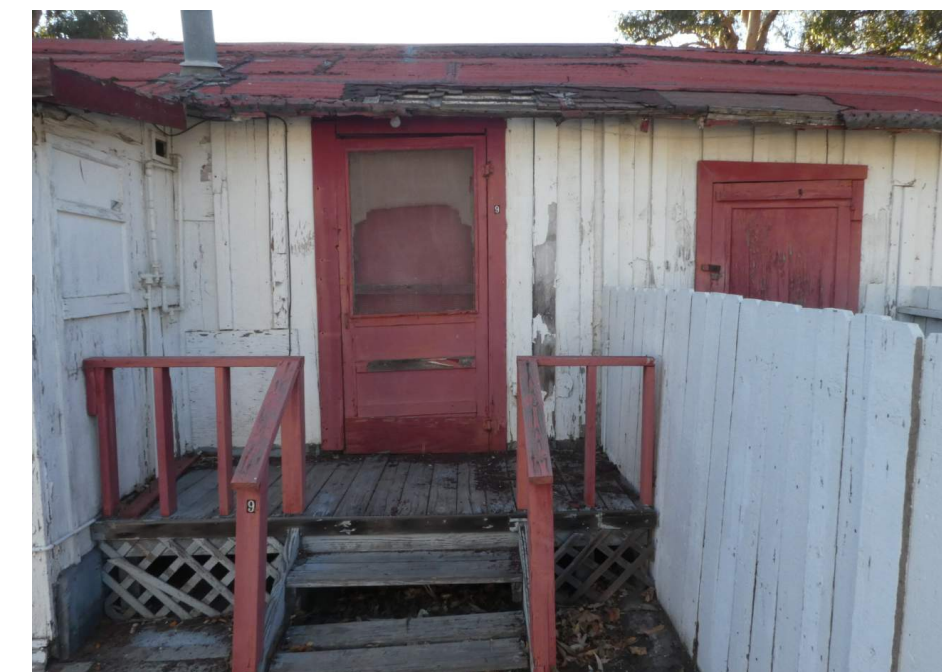
6 Unit 9 East Elevation
