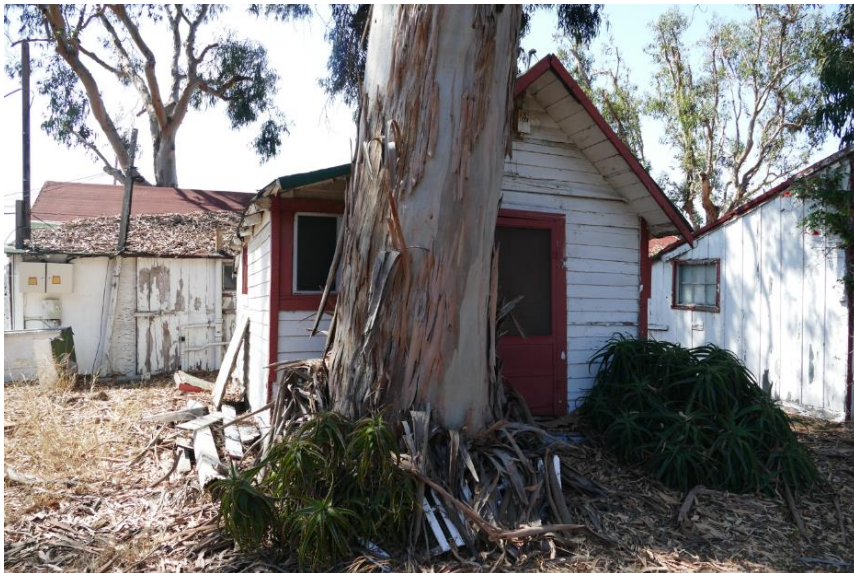
Figure 44. North elevation of Unit 21. Photo taken facing south.
