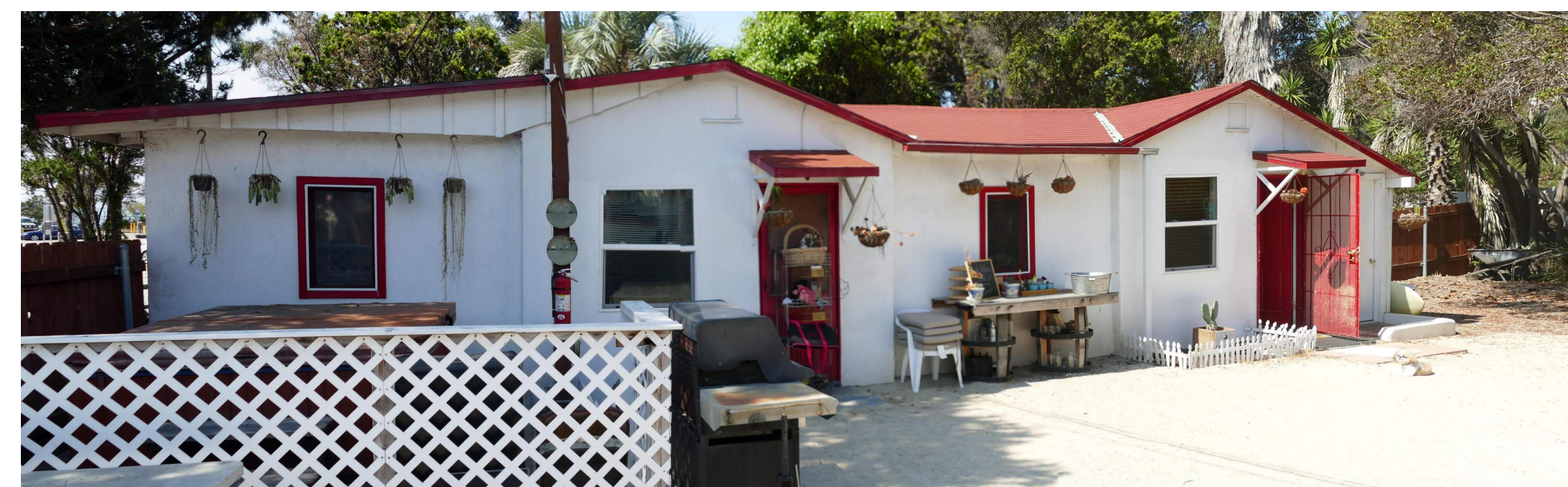
2 Cabin 16 North Elevation
