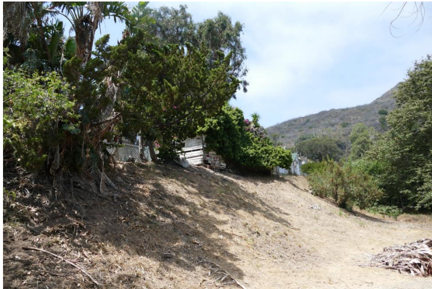
Figure 12. Sloped embankment of earthen fill located along the northeastern boundary of the site. Photo taken from the adjacent, lower flood plain area facing northwest.
