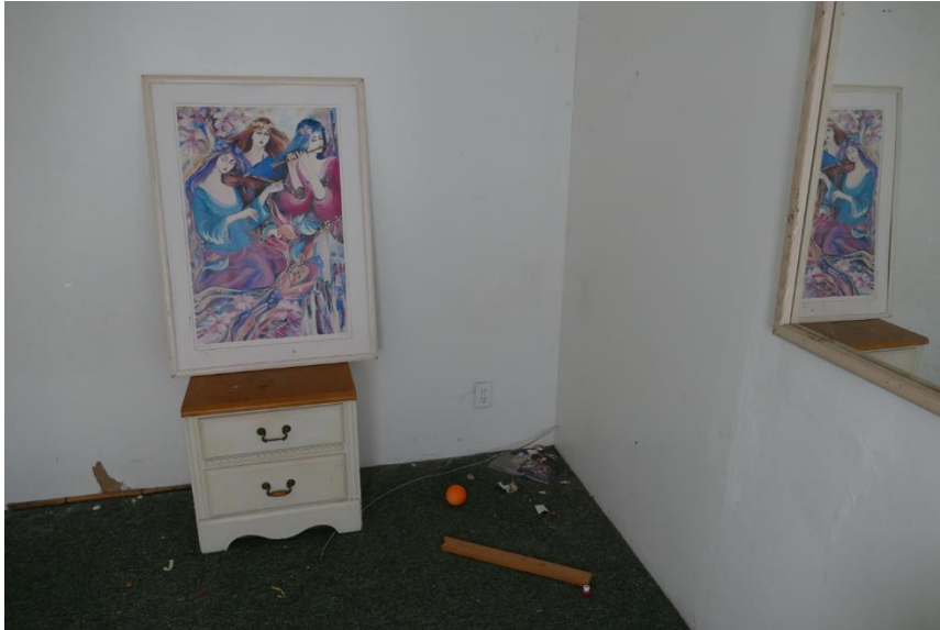
Figure 65. Typical interior gypsum board finish. Photo taken facing north in Unit 14.
