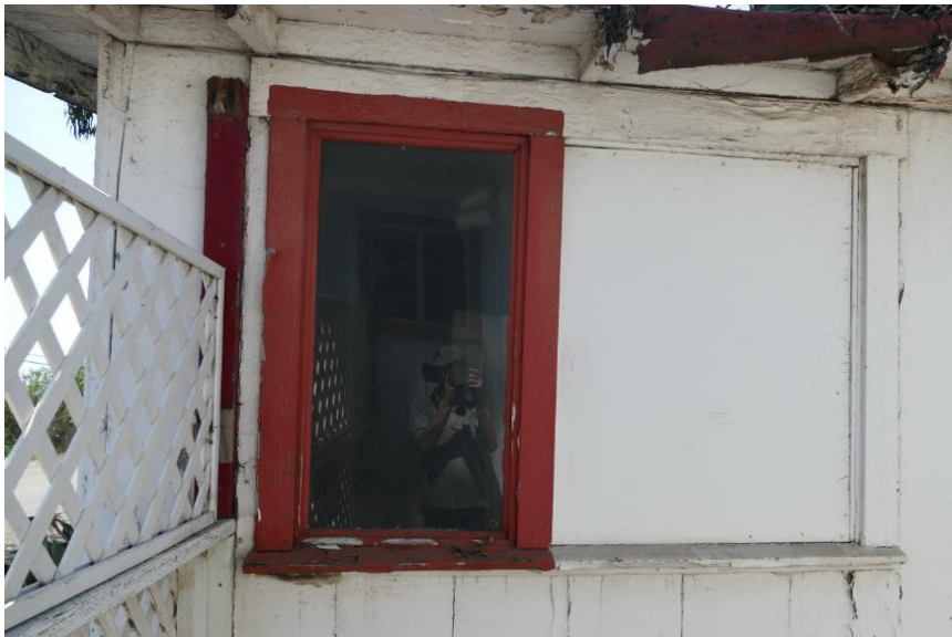
Figure 58. Typical single-lite fixed wood window. Photo taken facing southwest at Unit 2.
