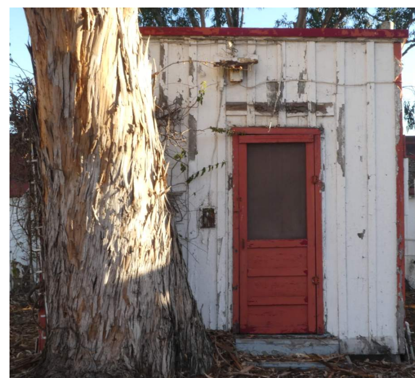
2 Unit 19 North Elevation
