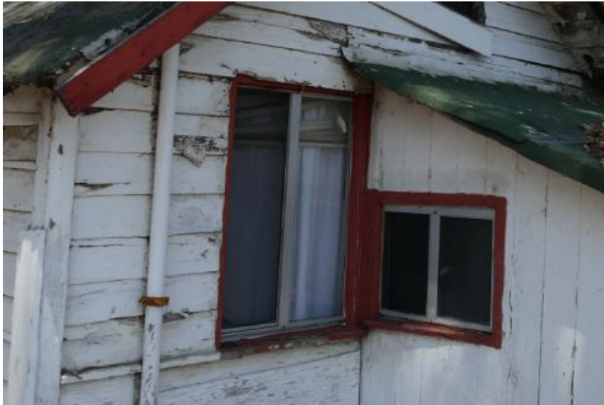
Figure 61. Typical single-pane sliding aluminum windows. Photo taken facing northeast at Unit 21.
