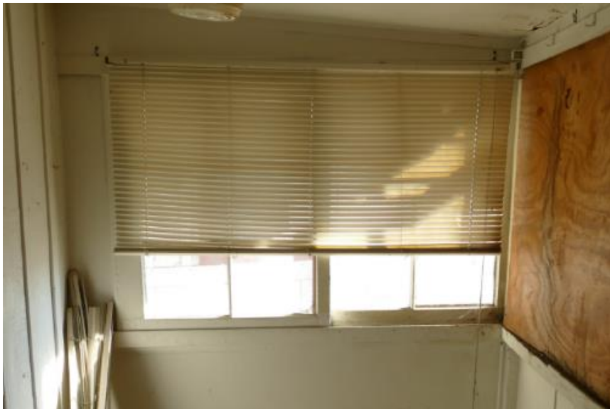
Figure 60. Typical sliding wood window. Photo taken facing east at Unit 1.
