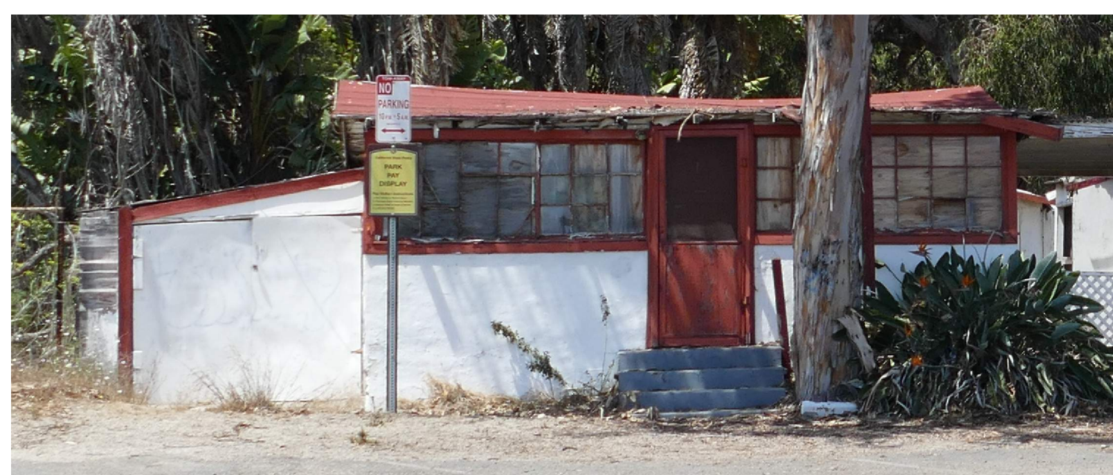
3 Unit 1 South Elevation
