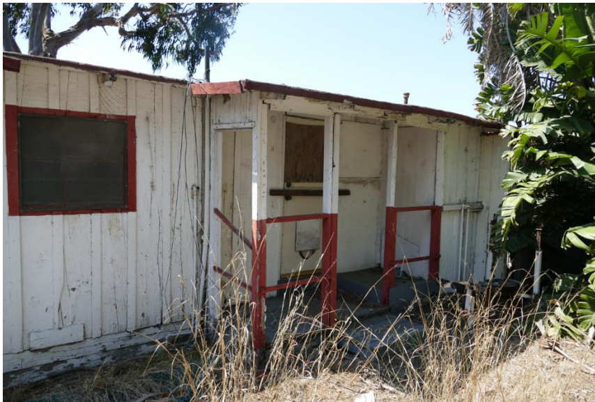
Figure 38. Covered entry porch at north side of Unit 1. Photo taken facing south.
