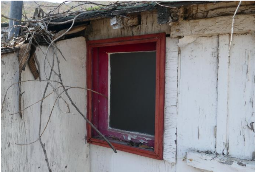
Figure 59. Typical casement wood window. Photo taken facing west at Unit 19.
