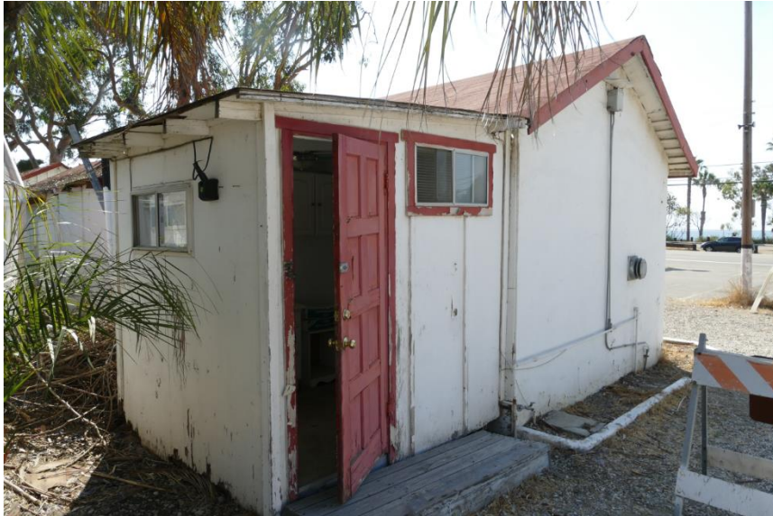
Figure 43. Northwest (rear) entry to the Office. Photo taken facing southeast.
