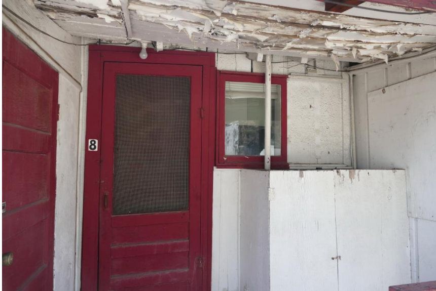
Figure 63. Typical wood screen door. Photo taken facing northwest at Unit 8.
