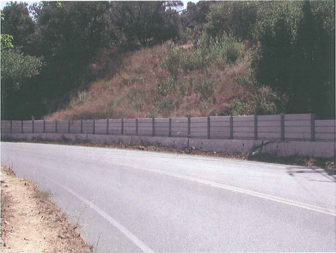
Figure 15 – View of Concrete Barrier Wall
