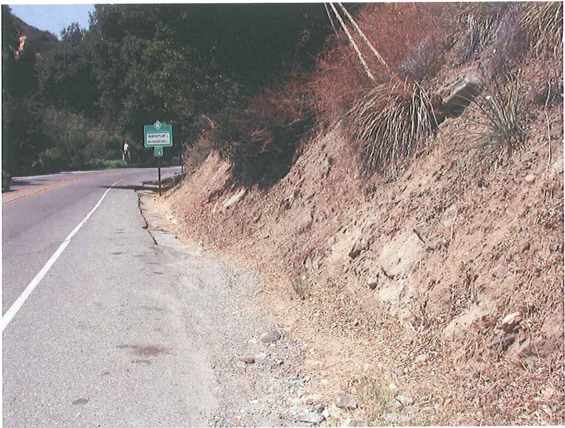
Figure 27 – Slope Mowing along SR-27
