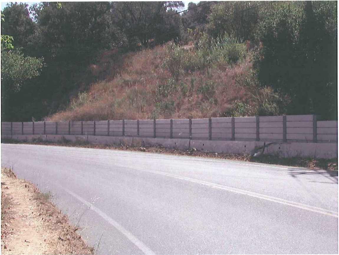
Figure 31 – Concrete Retaining Wall at PM 5.45
