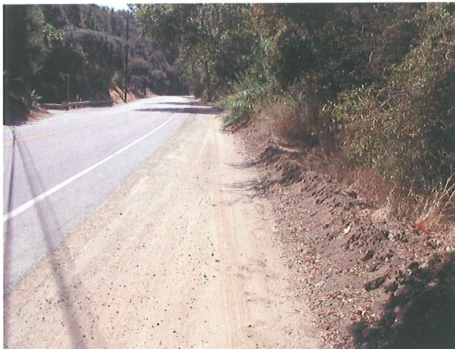
Figure 13 – Soil Berms along SR-27
