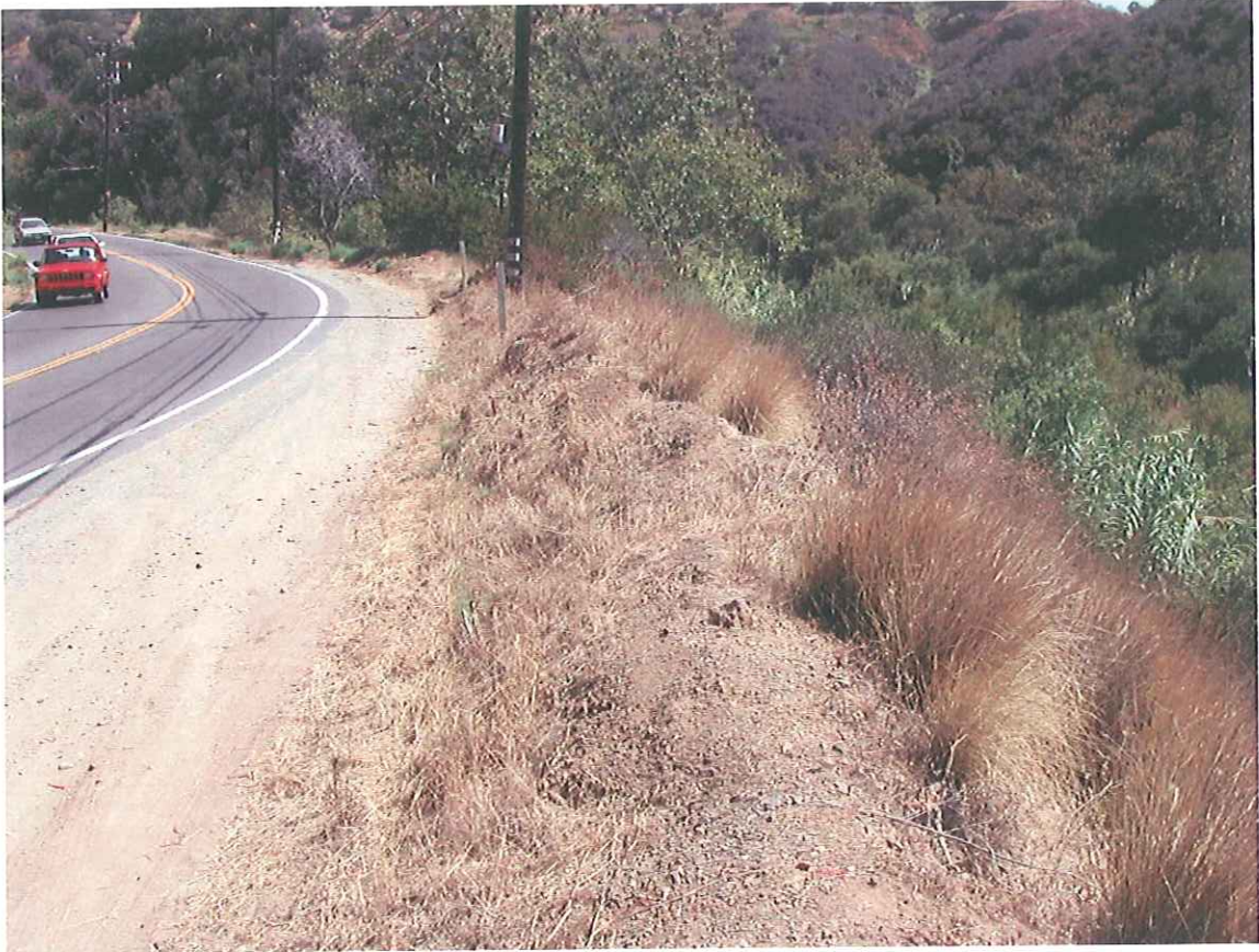
Figure 3 – Soil Berms along SR-27 adjacent to Topanga Creek
