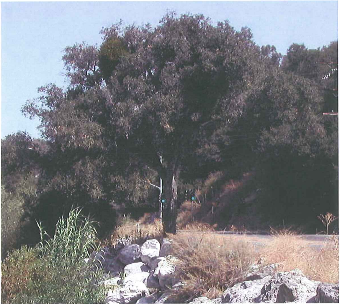
Figure 32 – Riprap Placed at Base of Oak Tree
