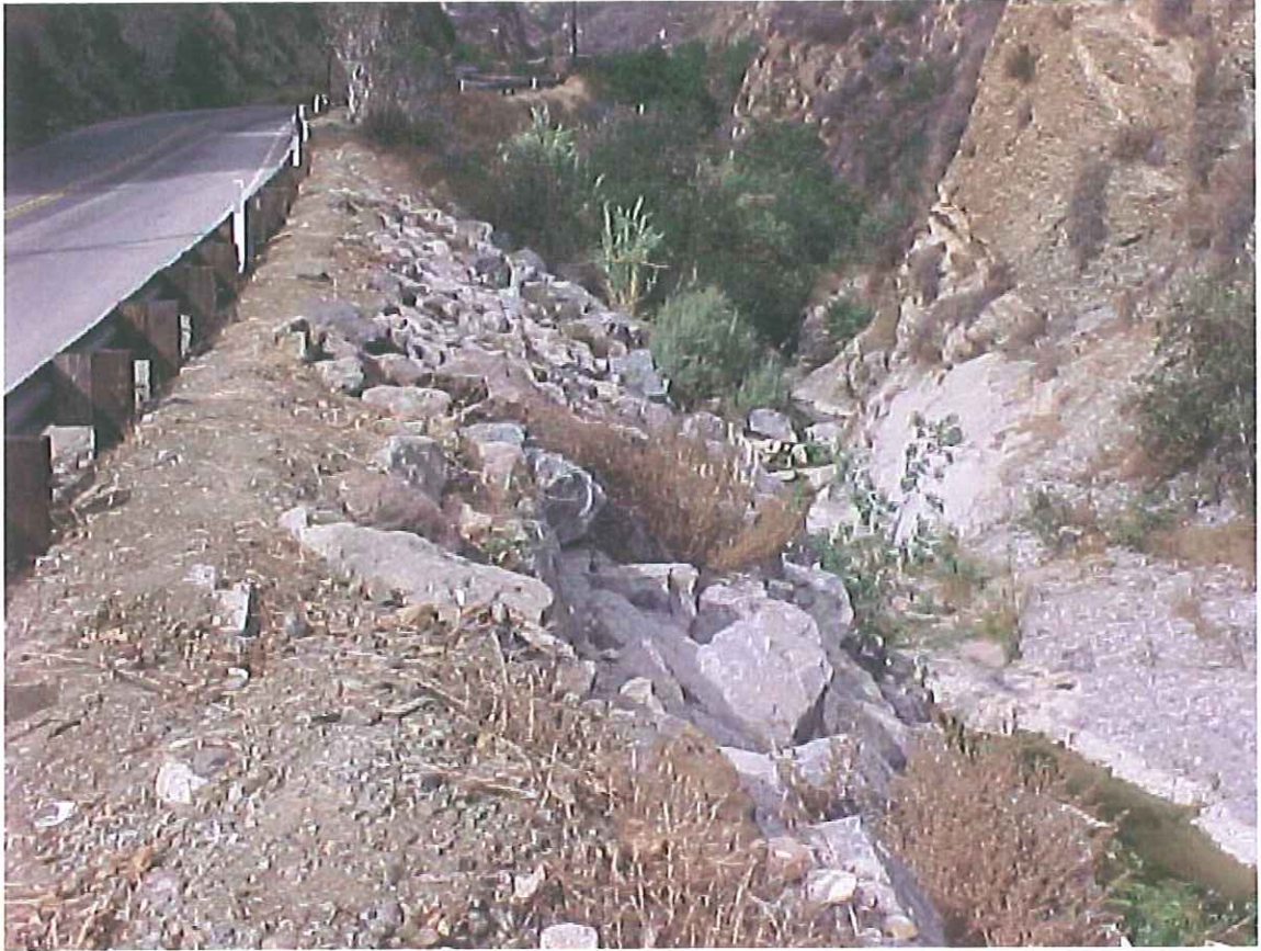
Figure 33 – Riprap on Slope adjacent to Steelhead Trout Location
