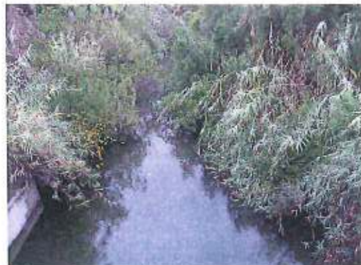
View from north side PCH bridge
