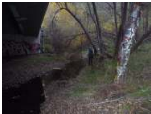
Topanga Bridge - 3600 m
