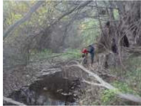
Topanga Bridge - 3600 m
